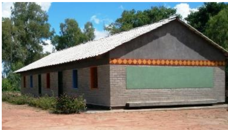
Figure 3: A newly constructed classroom block at Duma Primary
